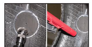
Use a soft wire brush followed by a vacuum to remove buffing dust and debris from the buffed area.
