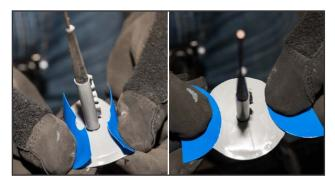
**13.** Reposition the poly on the cap to prevent contamination of the gray gum and allow easier removal of trapped air during installation.
