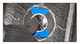
**16.** Press down the repair with your thumb from the center out.
