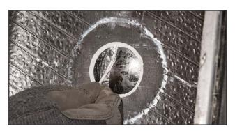
**19.** Remove the clear protective poly from the top of the repair.
