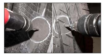
**6.** Damaged rubber and steel should be removed from the injury using a carbide cutter on a low speed air/electric drill, maximum 1,200 rpm. Drill the injury from the inside of the tire 3 to 5 times, followed by 3 to 5 times from the outside. In passenger tires, drilling the injury can be done with a 2,500 rpm air buffer as long as care is taken not to scorch the injury channel.
