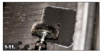
Clean the buffed area using a soft wire brush on a low speed buffer. Remove buffing dust by lightly brushing from the right side of the buffed surface to the left side. Repeat until all dust is removed.
