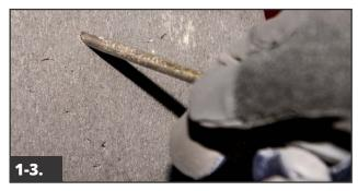
Using a probe, determine the size and angle of the injury while checking for rust and/or separation.
