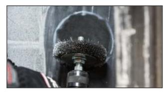
**11.** Clean the buffed area using a soft wire brush on a low RPM buffer. Remove buffing dust by lightly brushing from the right side of the buffed surface to the left side. Repeat until all dust is removed.
