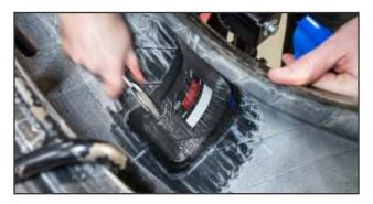
**20.** Remove the remainder of the blue poly from under the repair unit. As the poly is removed, press down the repair.
