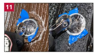
Stitch the repair from the center out. Remove the blue poly and stitch in the opposite direction.
