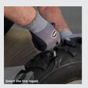
**Step 3:** Firmly press the repair into the puncture and pull insert tool straight back out.
