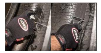
**3.** Place the tire so the repair area is in a 5 or 7 o'clock position to allow the buffing dust to fall to the bottom of the tire. Where permitted, the area can be cleaned by using CLC-704 Liquid Rubber Buff, to prevent contamination of tools. Use a scraper tool to remove contaminants. Repeat this process 2 or 3 times until all contaminants have been removed from the repair area.
