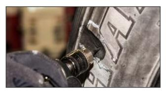
**6.** Remove all damaged steel at a 90° angle to the tire using a high RPM buffer (min. 20,000 rpm). Steel cables must be cut back into solid rubber. Inspect the area once the damage has been removed to assure that no damaged steel, splits, separations or rust remains in the tire.
