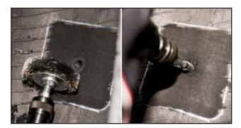
**11.** Clean the buffed area using a soft wire brush on a low RPM buffer. Remove buffing dust by lightly brushing from the right side of the buffed surface to the left side. Repeat until all dust is removed.
