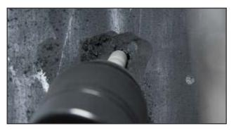
**6.** If cable damage is detected, use a pencil stone on a high-speed air tool (minimum 20,000 rpm) to dress cables into solid rubber. Care must be taken so that scorching of the rubber does not occur.
