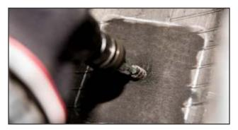
**7.** If a pencil stone was used, and/or scorched rubber is present, use a soft wire skive brush on a low rpm buffer to remove scorch without exposing steel cables.
