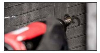
8. Remove any scorched or burned rubber using a soft wire skive brush on a low RPM buffer.
