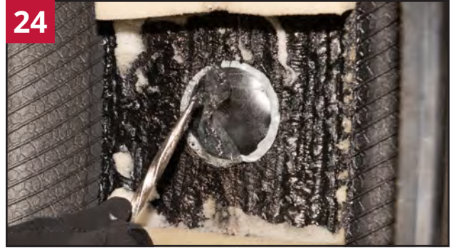
Remove the clear poly from the top of the repair unit.
