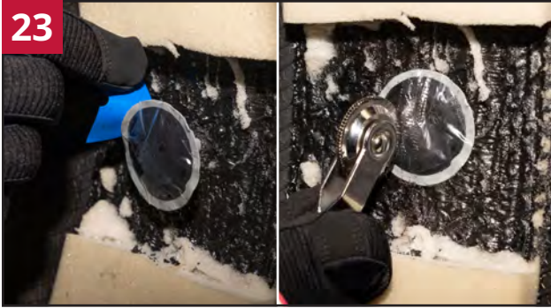
Remove the blue poly backing from under the repair unit and stitch the repair from the center out using firm pressure.
